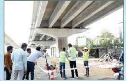
Bridge & Slab Load Test
