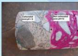
Carbonation of Concrete
